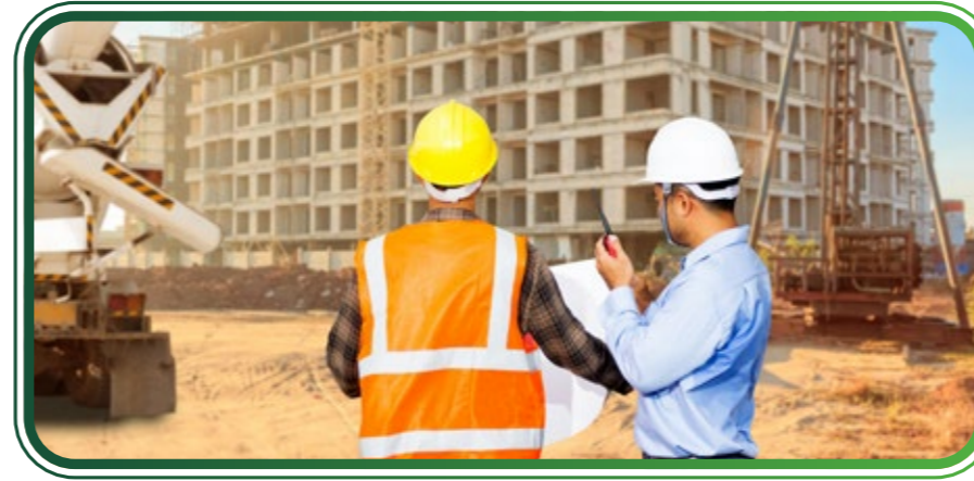
Health, Safety & Environment: Training local workforce to work in a safe environment including Safety gear usage, planning ahead, and risks assessment at work.
